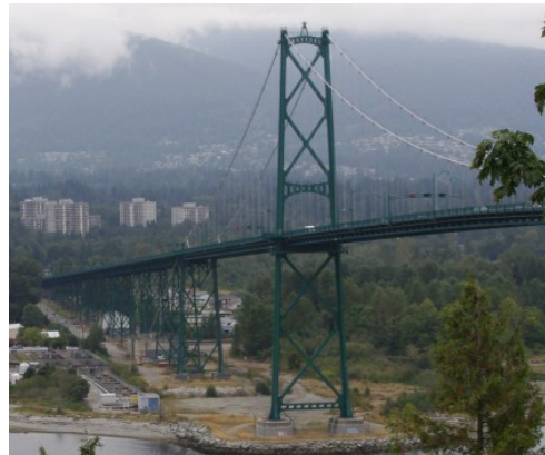
Bridge at Vancouver
